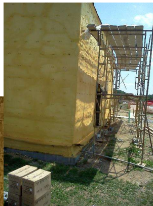
CI/WRB/AB on school (masonry cavity wall)
