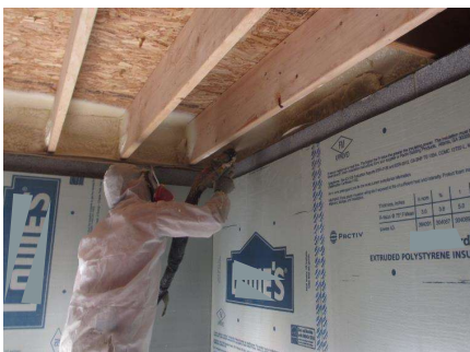
Air sealing & insulation for floor perimeter
