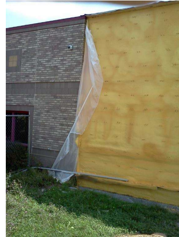
School Addition – Masonry/SPF/Brick cavity wall
